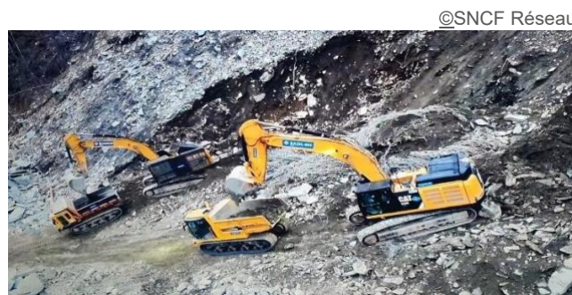
Clearing the gallery using radio-controlled machines
