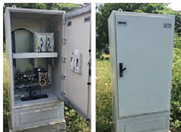
Lineside rack for peripheral interface components of ERTMS/ETCS L1 with Radio Infill
